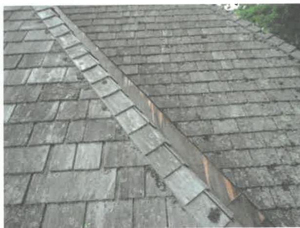
Figure 67 – West side roofing viewed from the north
