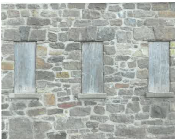
Figure 28- Covered windows, North wall
