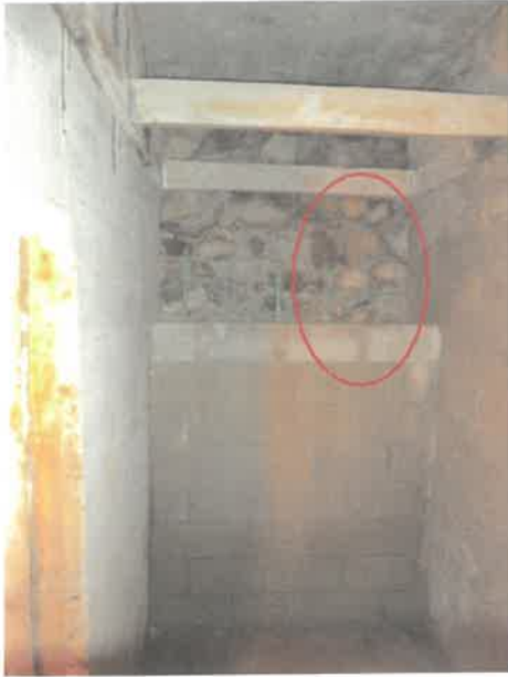
Figure 10 – North bracing wall
