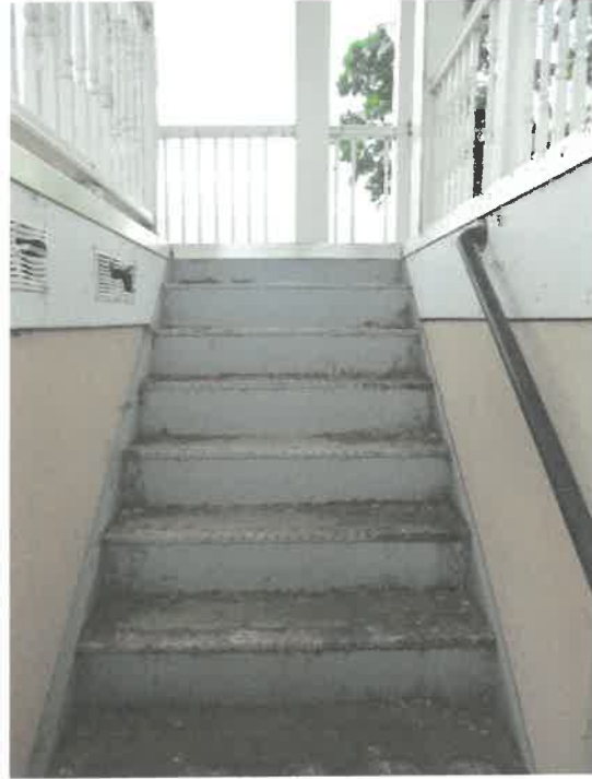
Figure 42 – Stair looking at Bandstand level
