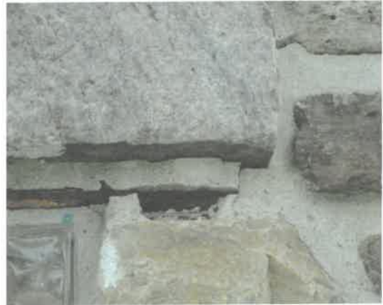
Figure 7 – West wall, Park level
