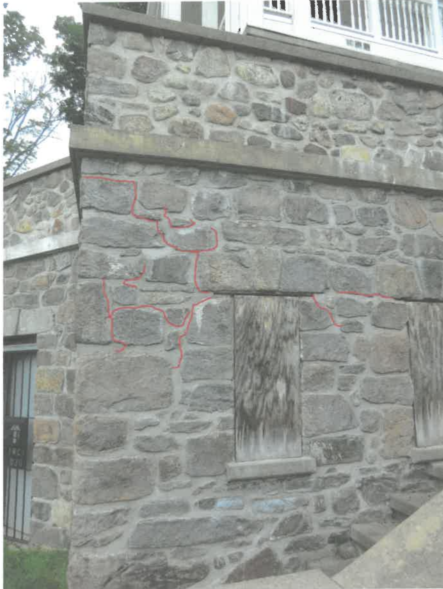
Figure 9 – SE corner of east wall at Bathhouse level
