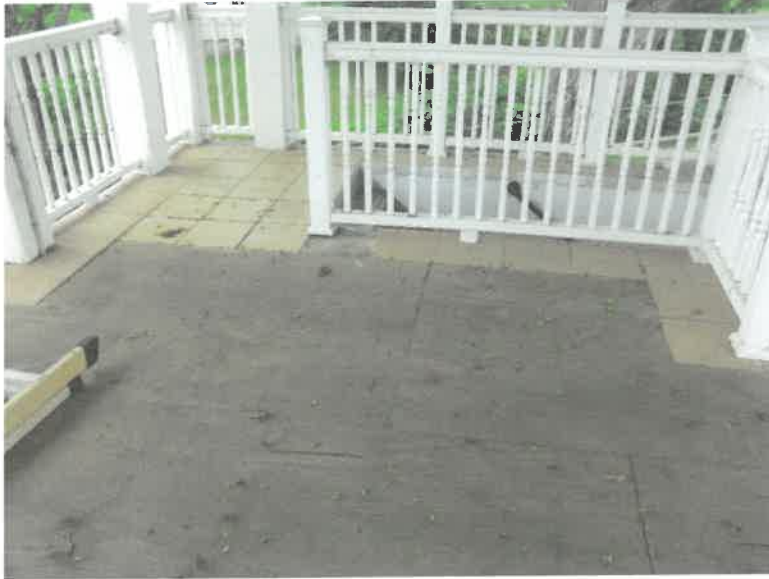
Figure 50 – West end including stairs
