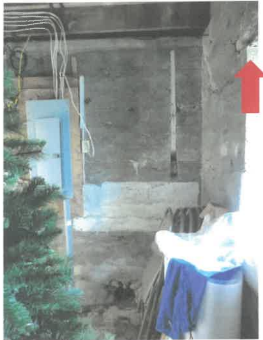
Figure 46 – North wall of Electrical room
