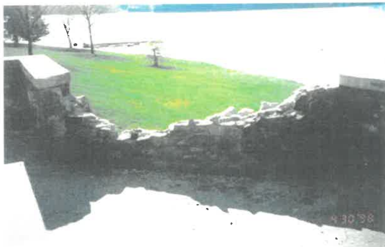
Figure 47 – 1998 Photograph of Terrace railing with concrete cap
