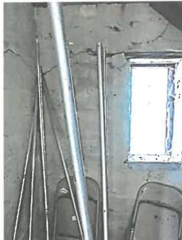
Figure 45 – West room, west wall
