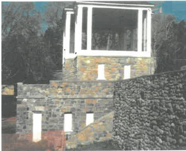
Figure 36 – 1999 Photo with windows covered
