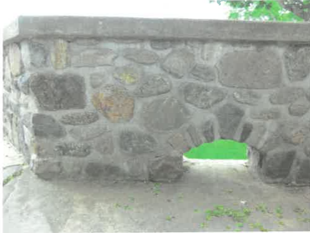
Figure 34 - Drainage opening for Park level slab
