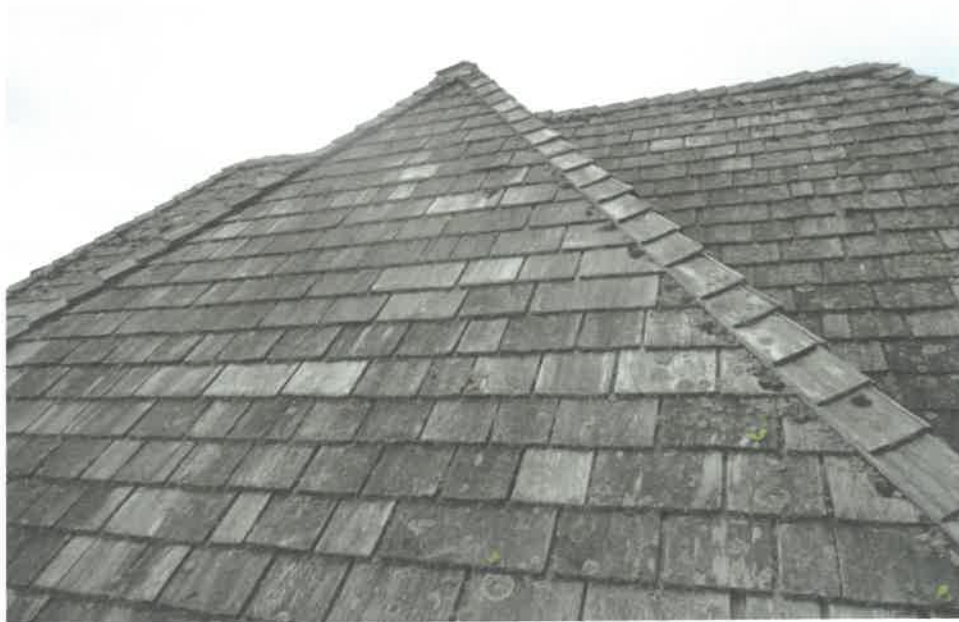
Figure 69 – West side roofing viewed from the north
