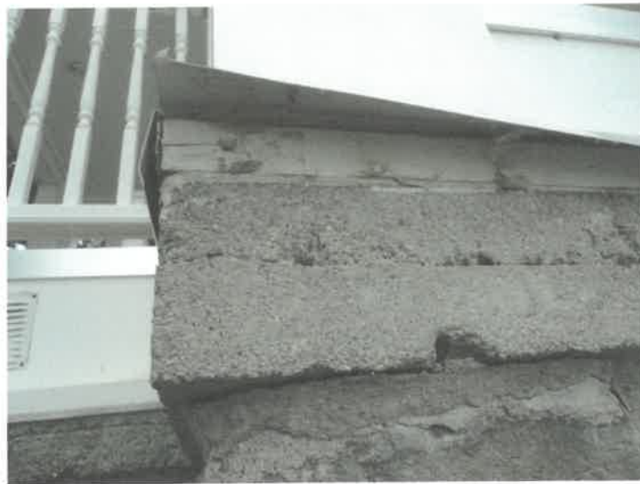
Figure 58 – Concrete cap on masonry pier with wood on top
