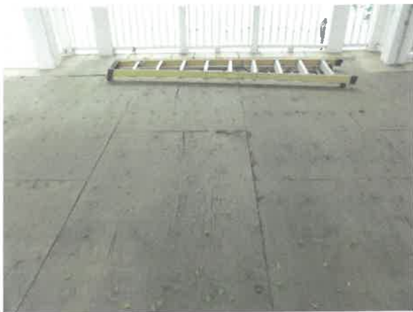
Figure 51 – Center of Bandstand floor
