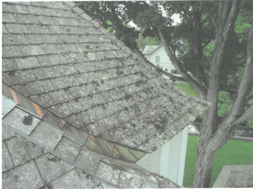
Figure 68 – West side roofing viewed from the north
