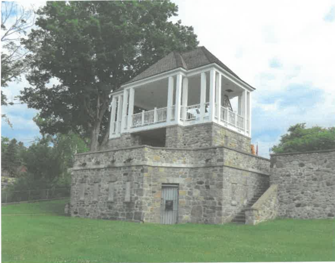
Figure 3 – View from southeast with Bathhouse at lowest level
