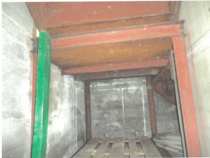
Figure 43 – Stair support in west side room
