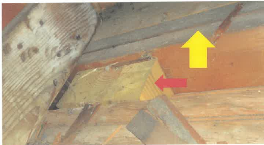
Figure 62 – Top of wood posts in the attic
