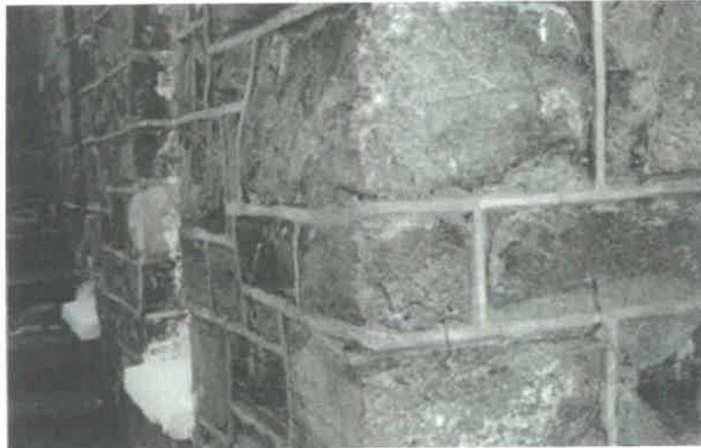
Figure 17 – Stonework before 1999 repairs
