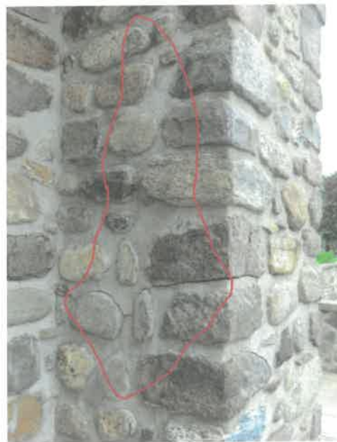
Figure 12 – NW pier at Park level
