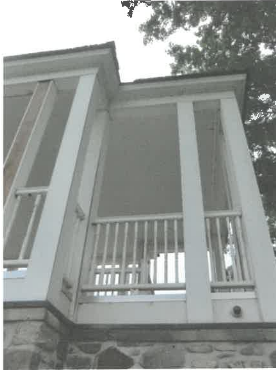
Figure 63 – Existing beams and columns without ornamentation
