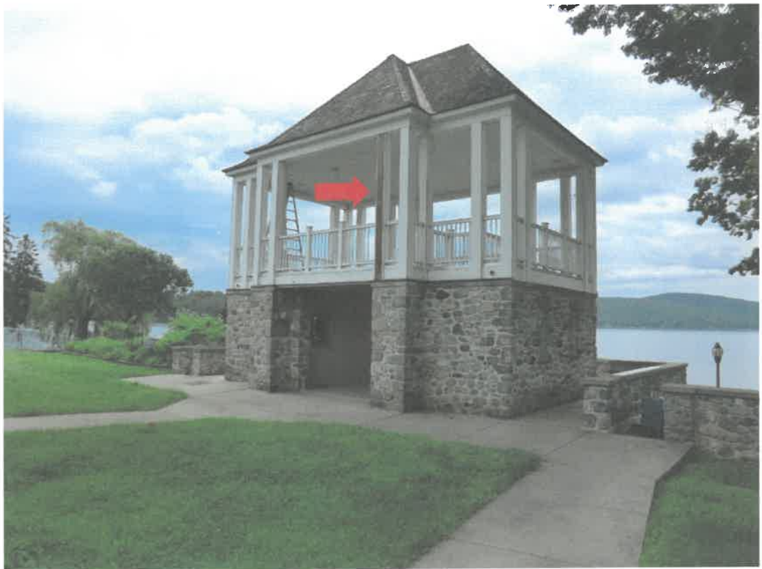
Figure 55 – Column post cover removed on a north column
