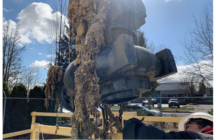
Wipes clogging a pump in a neighborhood in Vancouver, WA. Photo courtesy of the Association of Clean Water Agencies (ACWA).
