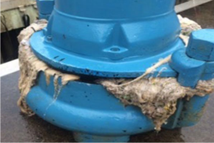
Wipes clogging a pump in a neighborhood in Vancouver, WA. Photo courtesy of the Association of Clean Water Agencies (ACWA).
